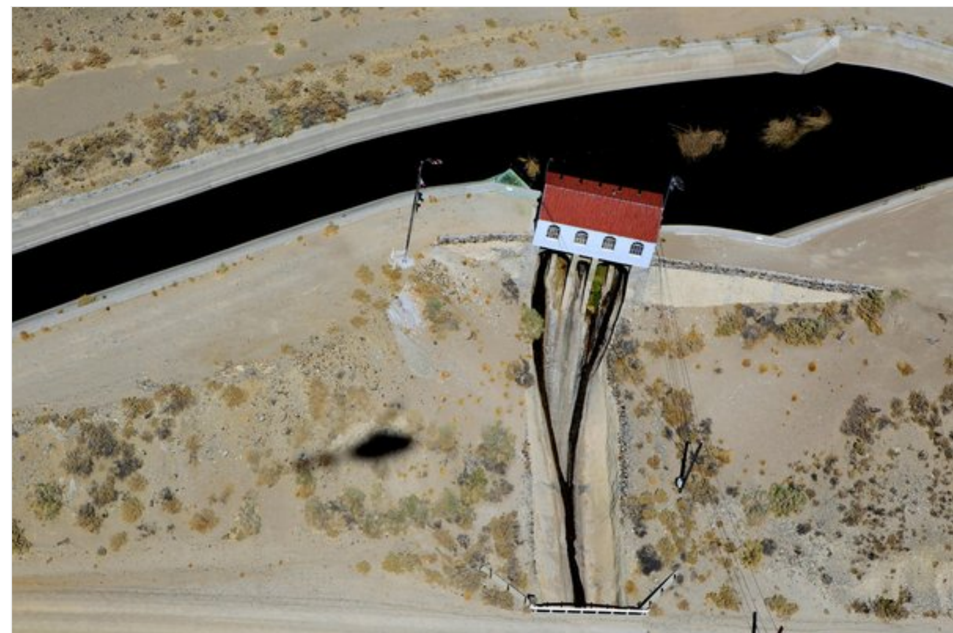
An aerial view of the Alabama Gates along the Los Angeles Aqueduct. A 1976 explosion ripped apart the steel gate, which regulates the flow of water to the aqueduct. About 100 million gallons of water meant for Los Angeles were instead flushed into Owens Lake. (Brian van der Brug /
