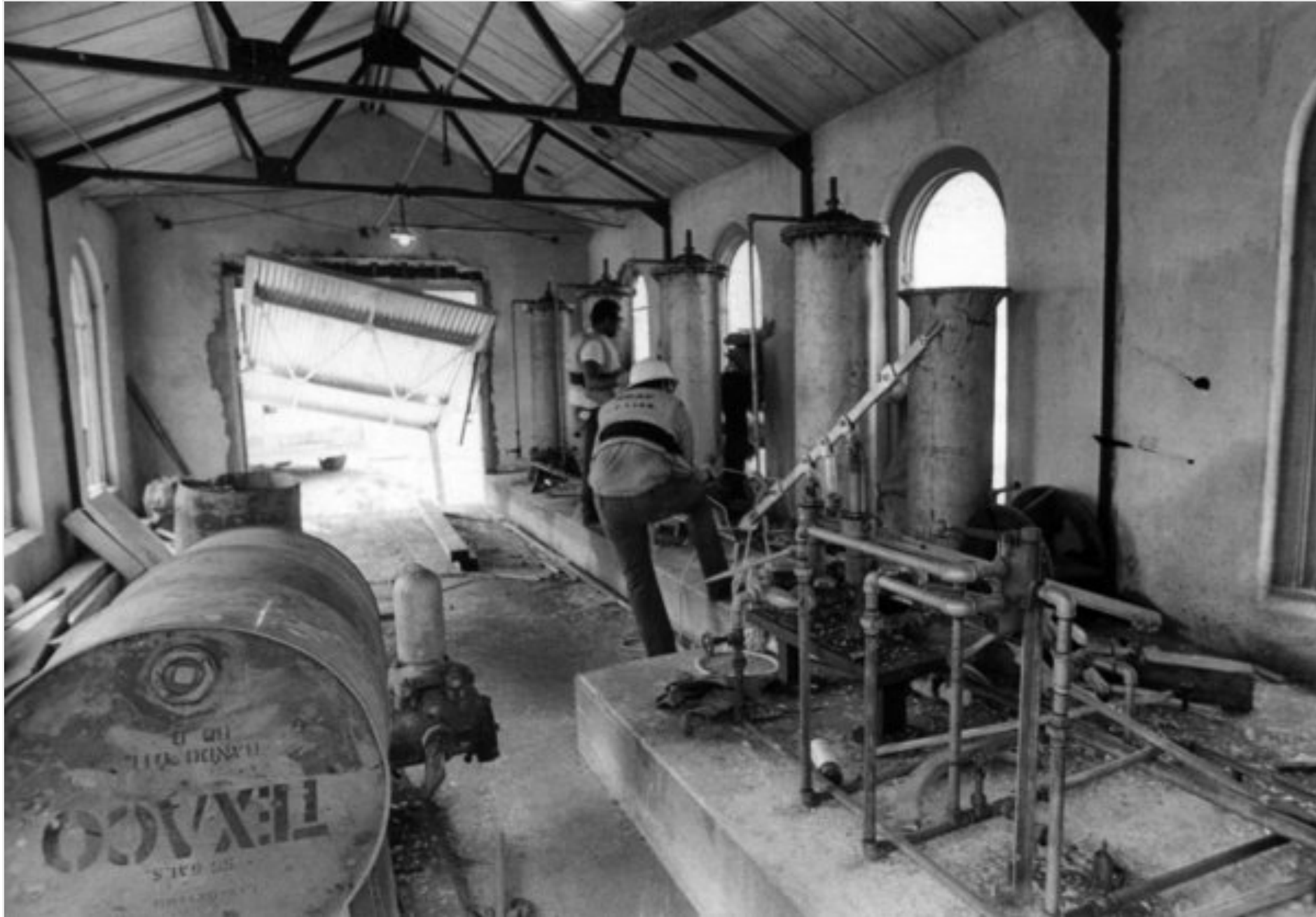
The interior of the Los Angeles Aqueduct's Alabama Hills gatehouse after an explosion buckled the floor and blew out the windows and door. This photo was published in the Los Angeles Times on Sept. 16, 1976. (Ben Olender) More photos
